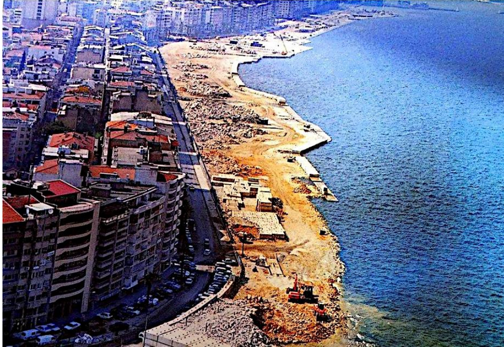
Figure 3. Land Reclamation in Kordonboyu in 1997 (Source: www.izmirmag.net )
