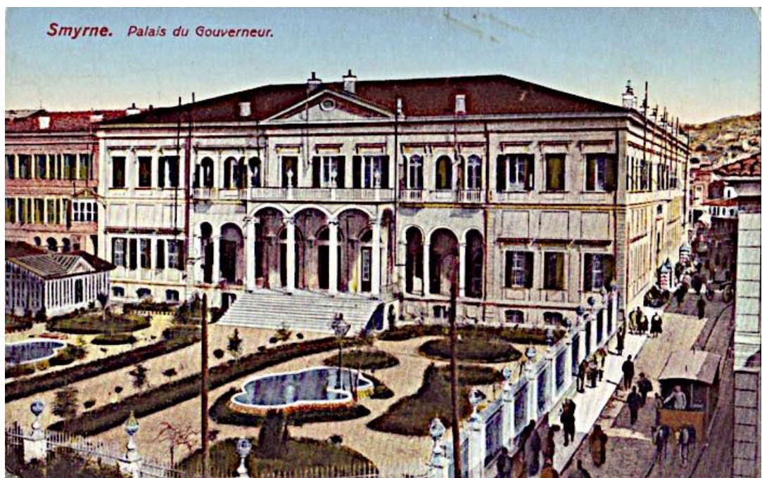
Fig. 4. Government House completed in 1872 [32]
