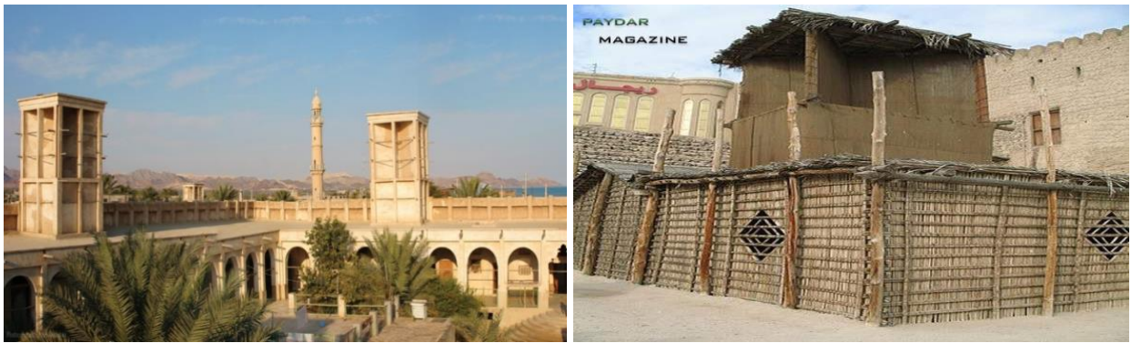
Fig. 9. Sample of hot and humid traditional houses structure (Hormozgan, Iran)
