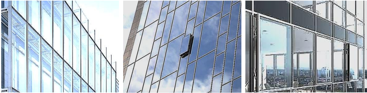
Fig. 5. Curtain wall facade
